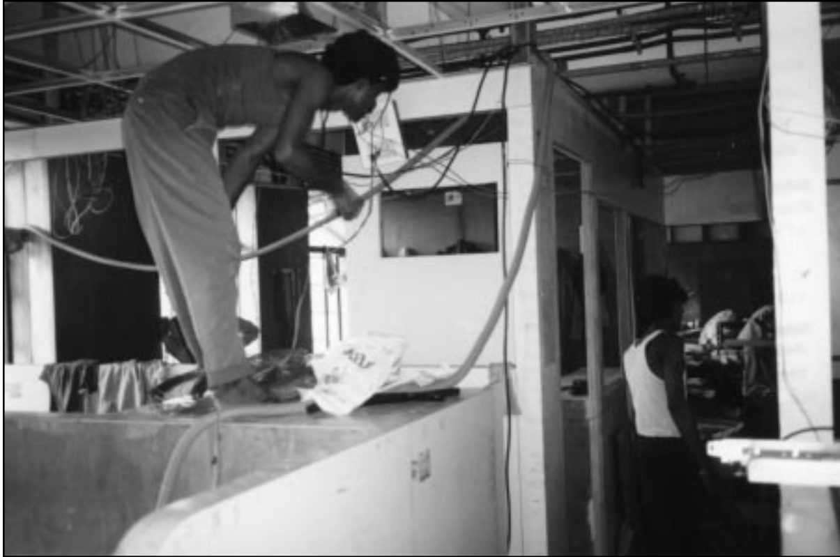
Figure 51 The Emergency Operations Center in Mantralaya under construction.
